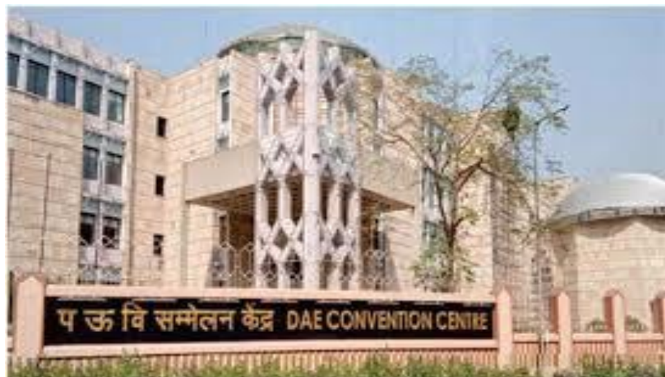
DAE Convention Centre at BARC, Mumbai
