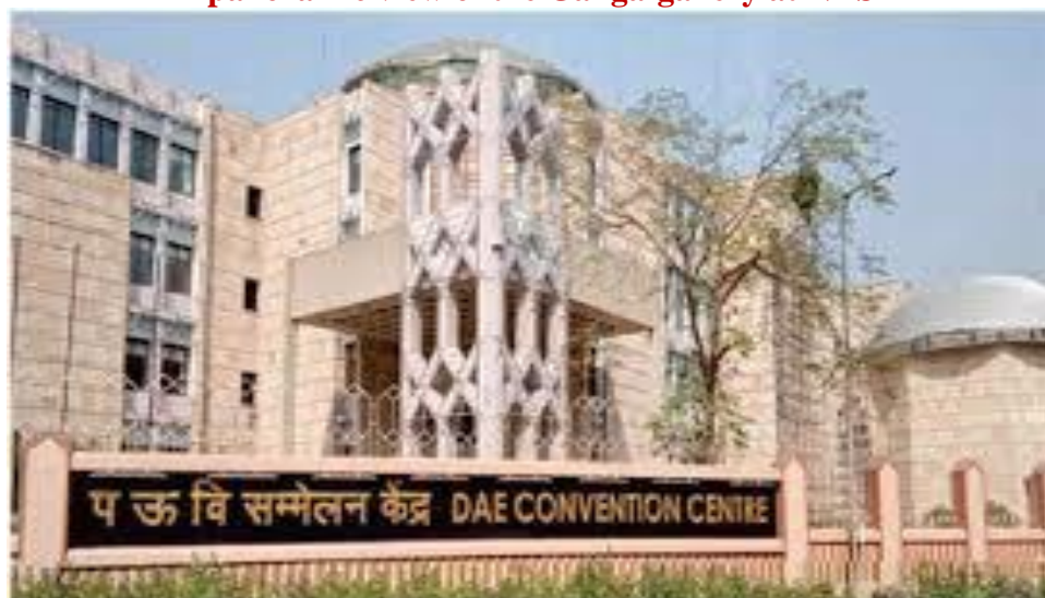
DAE Convention Centre at BARC, Mumbai
