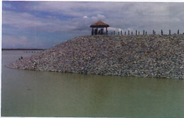
Embankments with boulder revetment
