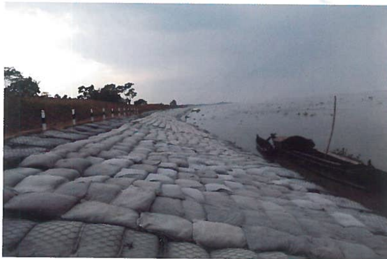
Embankments with slope protection using geo-bags
